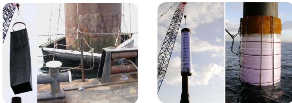
Figure 6.7 Rubber sleeve 3-6 mm thick typically used for airborne sound attenuation (left) and foam-coated steel sleeve (right). From Nehls et al., 2007.
