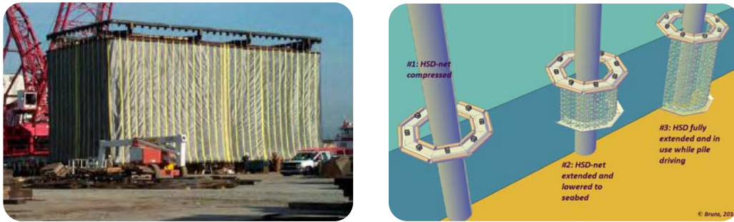
Figure 6.2 Photography of the confined air bubble curtain Gunderboom® out of water (left) and details of the deployment of a Hydro Sound Damper (right, from Bruns et al., 2014).
